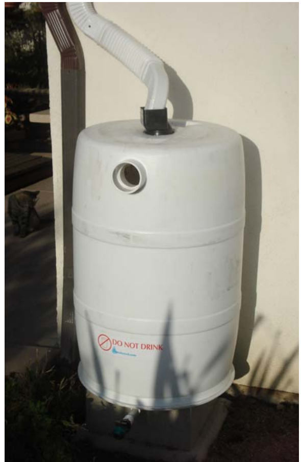
Rain barrels, like this one in my garden, are easy to install, conserve water and reduce coastal pollution.
